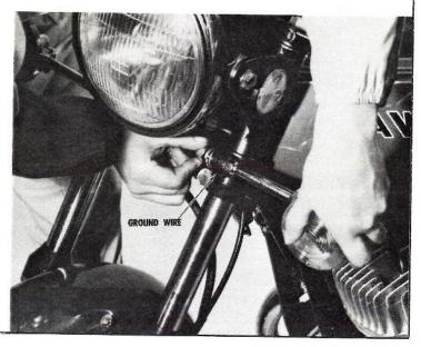
Mount the left rear turn signal. Be sure all the parts shown here are installed in the order shown below. NOTE: The ground clip must be fitted to grommet "A" or the lamp will not light.
